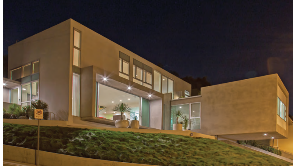
The Cantilever House :: leeMundwiler architects $2,495,000 2955 Swan Place, Silver Lake Brian Linder, AIA | 310.592.5417 William Baker | 310.867.0847
