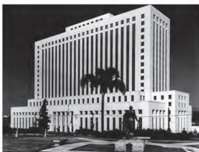
Federal Court House, LA – 1942
