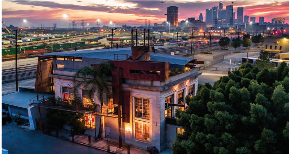
The Carlson-Reges Residence, 1922 698 Moulton Avenue, Los Angeles, CA 90031
