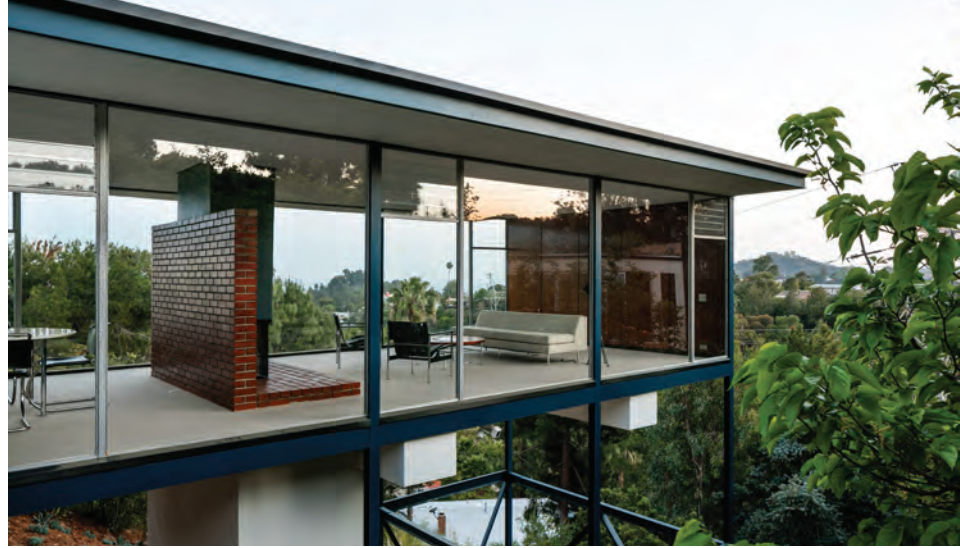
Craig Ellwood/James Tyler, FAIA, 1958/2018 1095 N Kenter Avenue, Crestwood Hills
